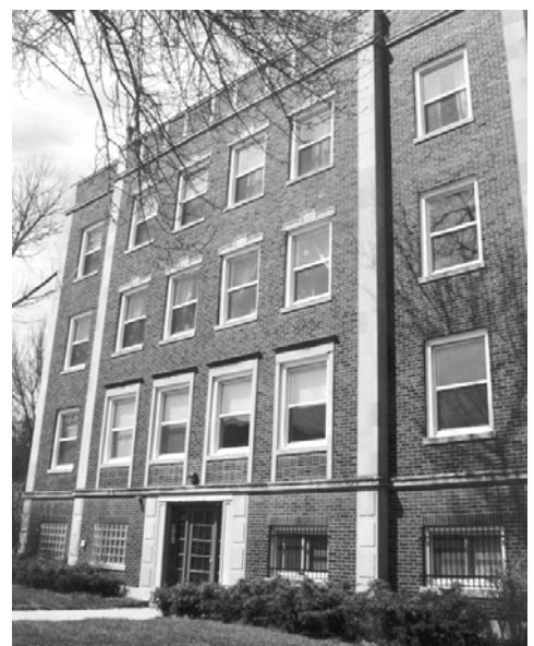
Project team seeks apartments like these owned by HODC
